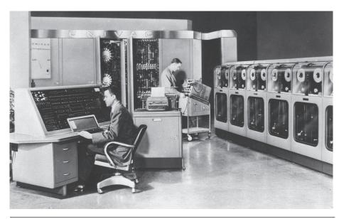
**FIGURE 1.12.2 UNIVAC I, the first commercial computer in the United States.** It correctly predicted the outcome of the 1952 presidential election, but its initial forecast was withheld from broadcast because experts doubted the use of such early results.
